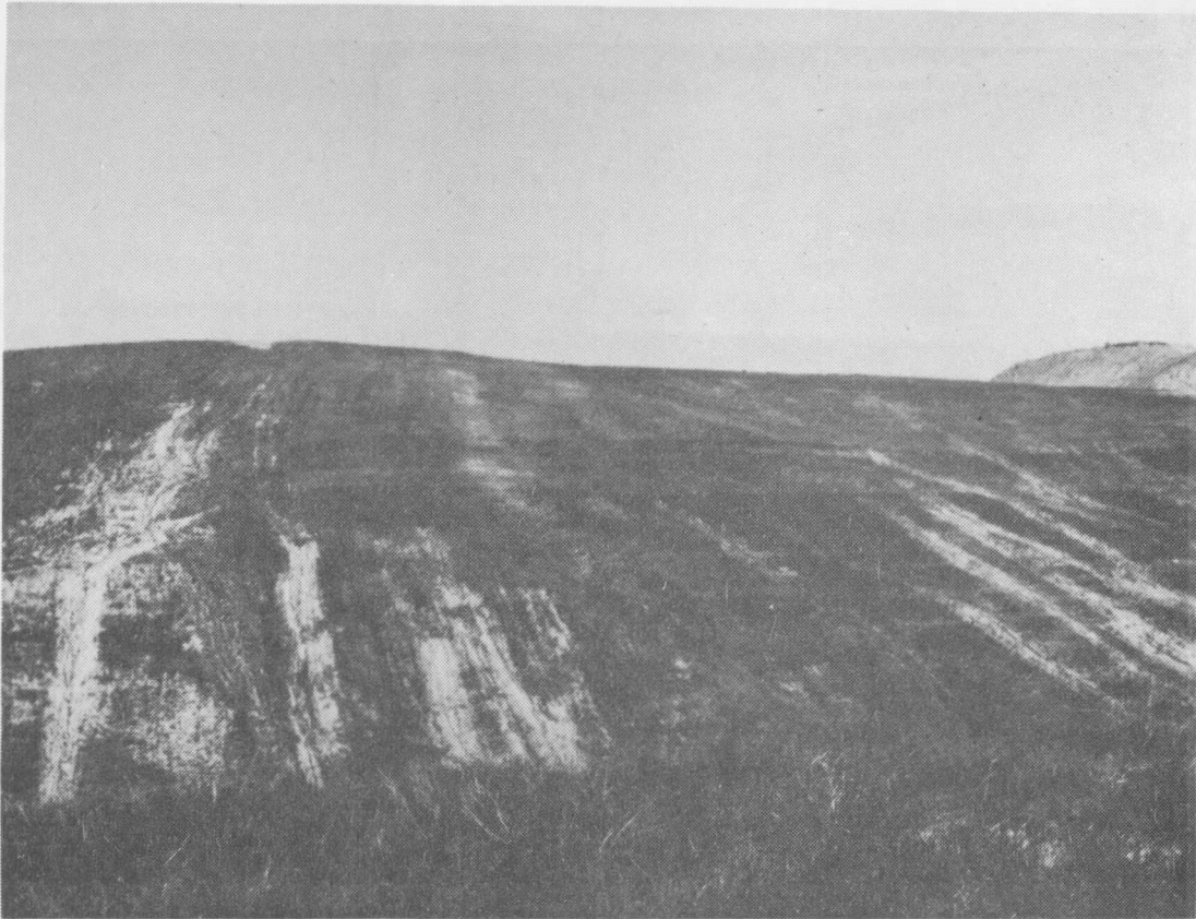
Figure 31. Head-cutting rills and gullies formed at the Westmoreland Mine as well as at other mines where long straight or convex slopes were created. Concave slopes which are often the equilibrium form in nature may be less susceptible to this kind of erosion.
