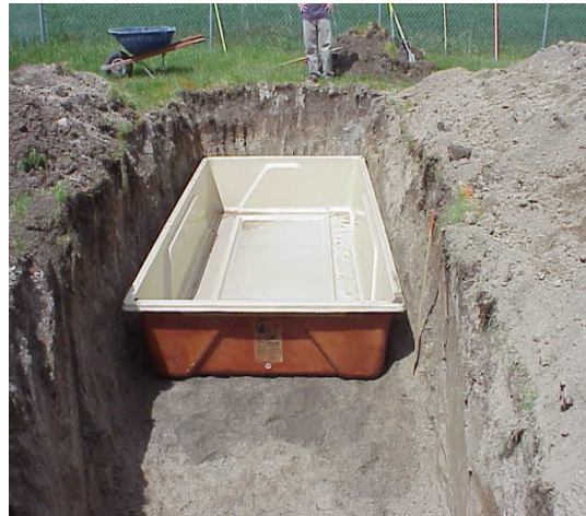
Figure 3.2: Fiberglass trough in bottom of excavation.
