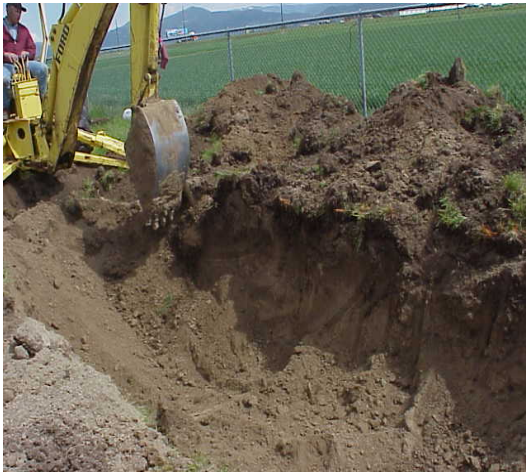
Figure 3.1: Excavation of field frost heave test facility.
