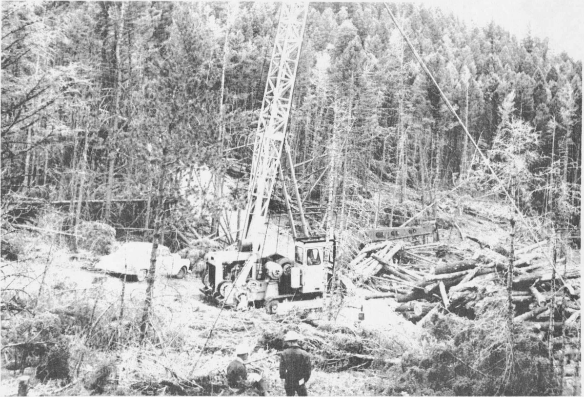
Figure 8. A Skagit system used for high lead skidding.
