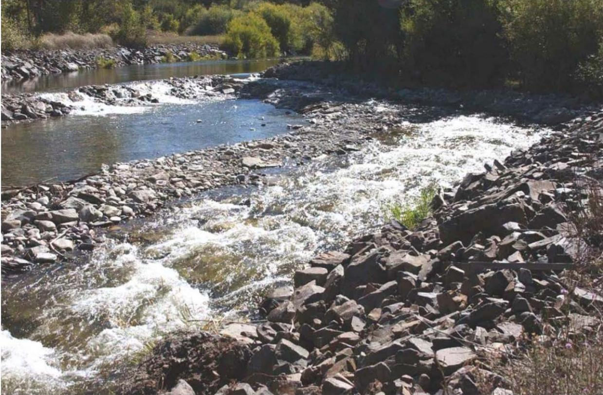
*Figure 18 - Example of a rocky ramp style fish way. Photo by USBR.*
