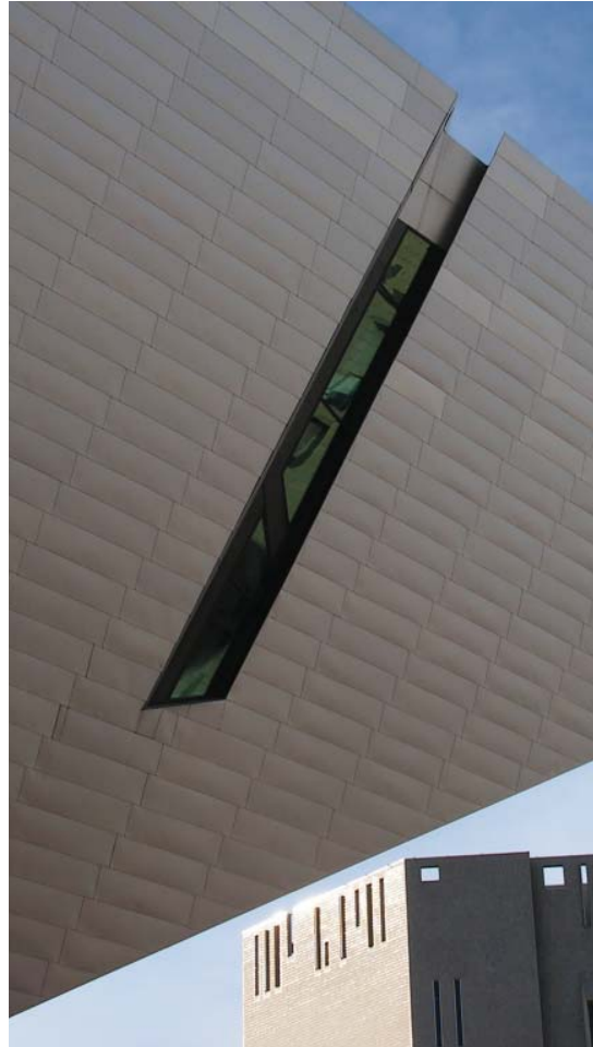
Image 35 - Outside view of the north leading edge.
