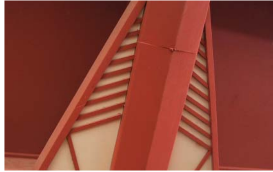
Image 31 - Roof detail, inside meeting room.
