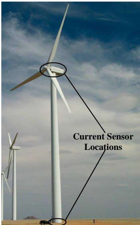
Figure 44: The base of the tower and the nacelle have many sensors, the blades, however, still have no sensors.
