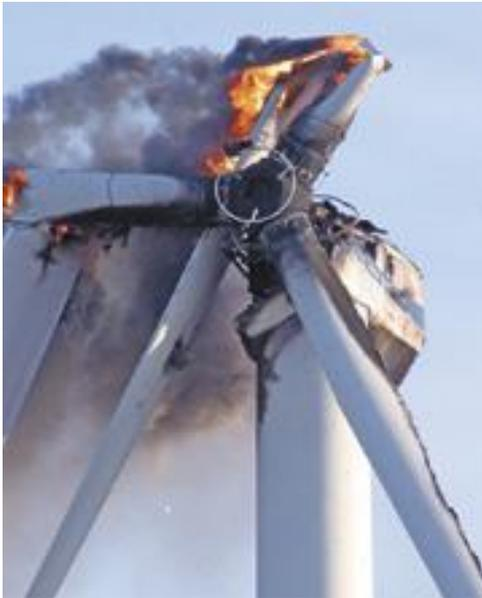
Figure 10: Without proper load control mechanisms severe damage and even destruction of a wind turbine can occur.
