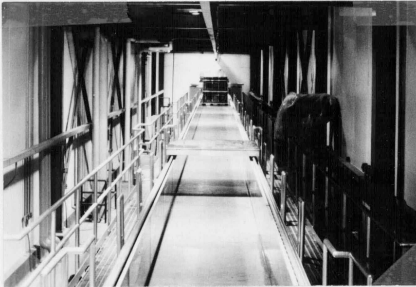
Figure 5. Photographs of Hydraulic Flume.
