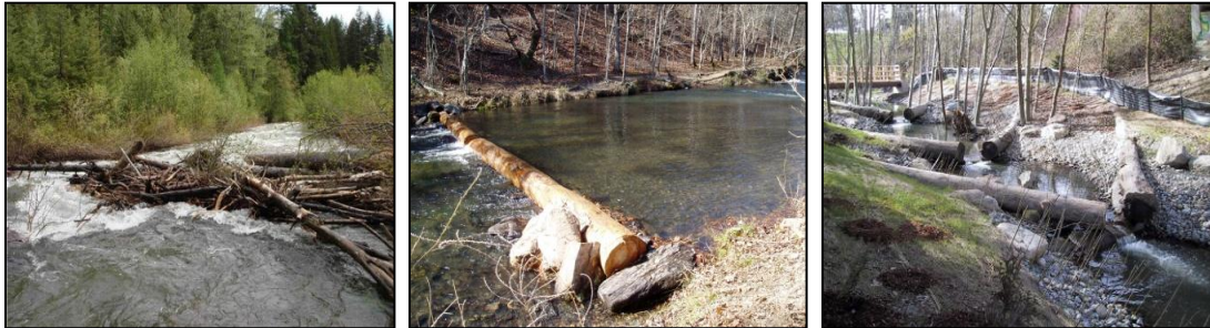
Figure 1. Examples of habitat enhancement structures. From left to right: Artificially constructed log jam (USFS), check dam structure (Oklahoma Department of Wildlife Conservation), and log cross vanes (National Center for Earth-Surface Dynamics).
