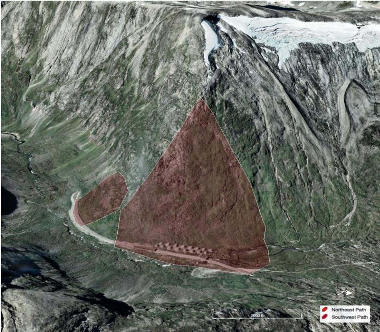
Figure 3. NE and SW slide path of Sætreskarsfjellet Mountain above highway 15 used in this study.
