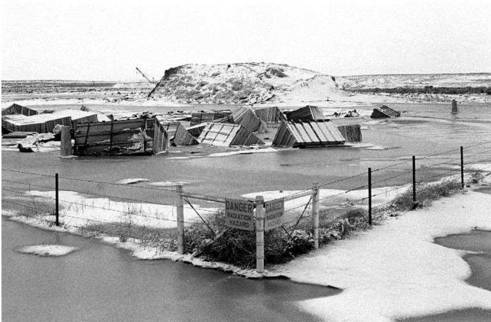
Figure 3: NRTS flooded pit no. 9, January 1969
