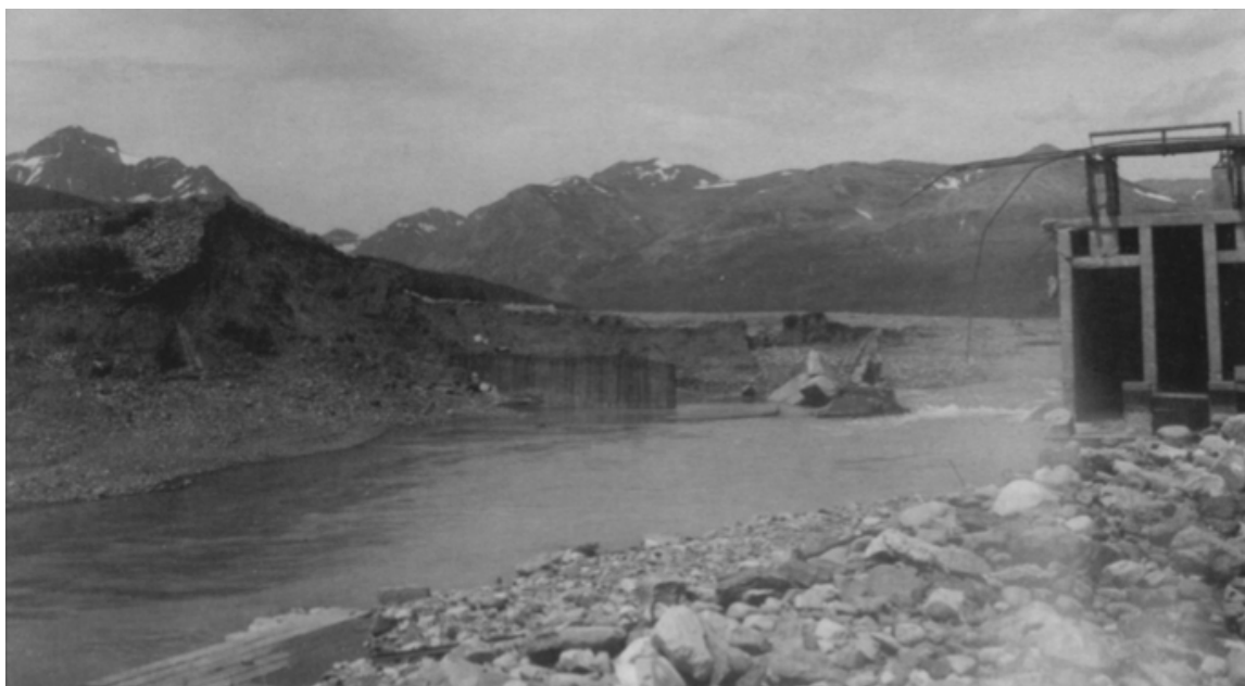
Figure 11. Two Medicine Dam, After.
