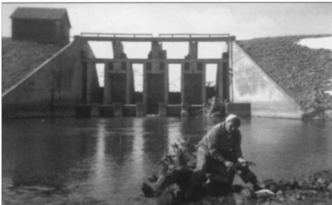
Figure 10. Two Medicine Dam, Before.
