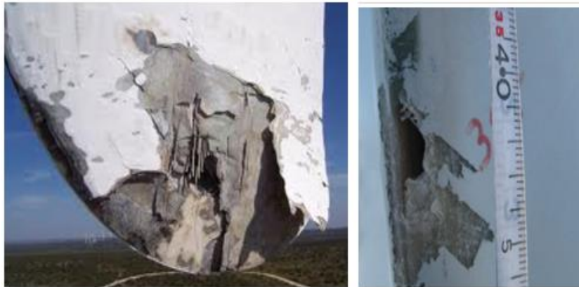
Figure 1: Wind Turbine Blade Damages
