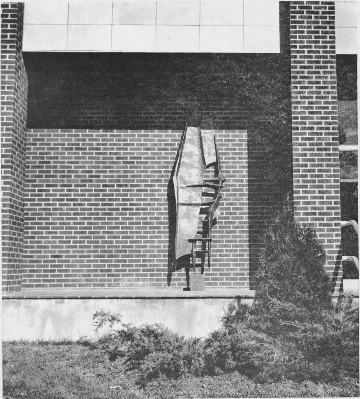
Figure 13 Completed Section at the Site
