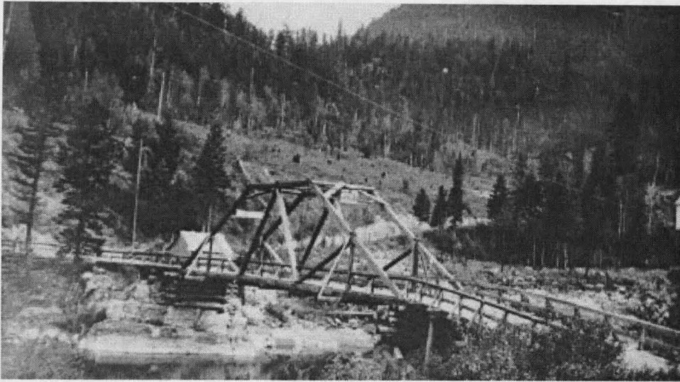
Figure 6. The First Middle Fork of the Flathead River Bridge
