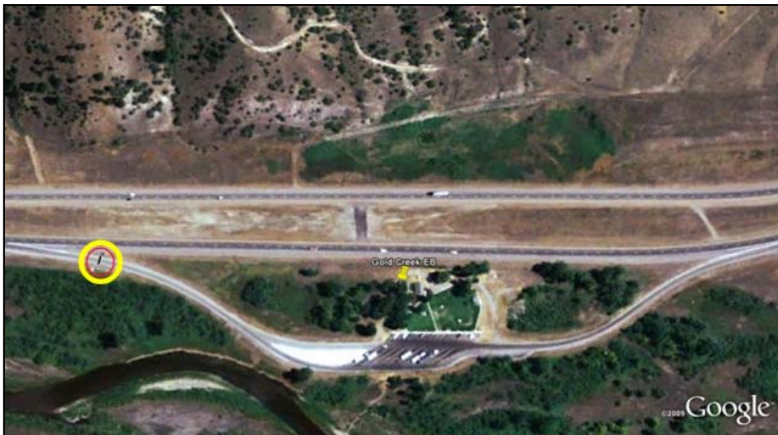
Figure 2: Setup Location for Sites with Typical Geometry - Gold Creek Eastbound Rest Area (Image Source - Google)
