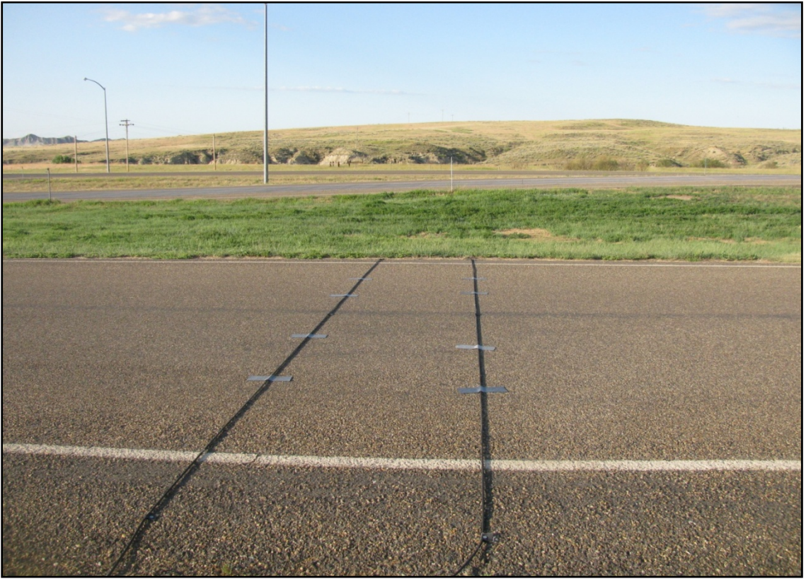
Figure 3: Pneumatic Tube Setup
