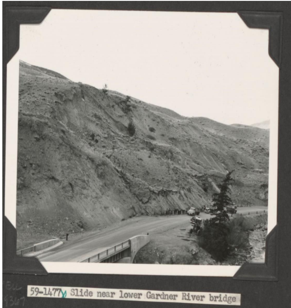
Figure 10B. Archived photo taken from Open Parks Network of a reactivation that occurred in 1959 on the toe of landslide 5.
