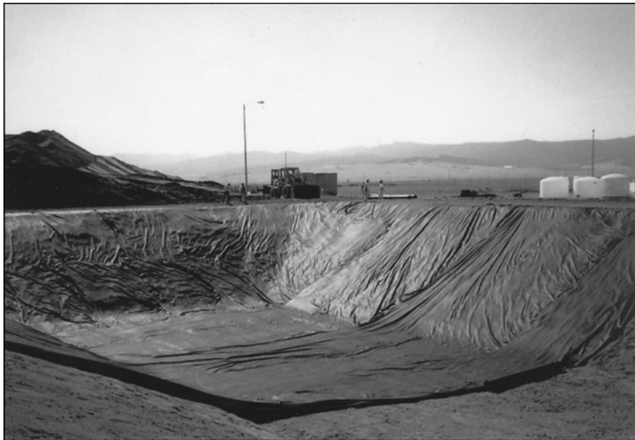
Figure 3. Test cell construction showing installation of the impermeable liner.
